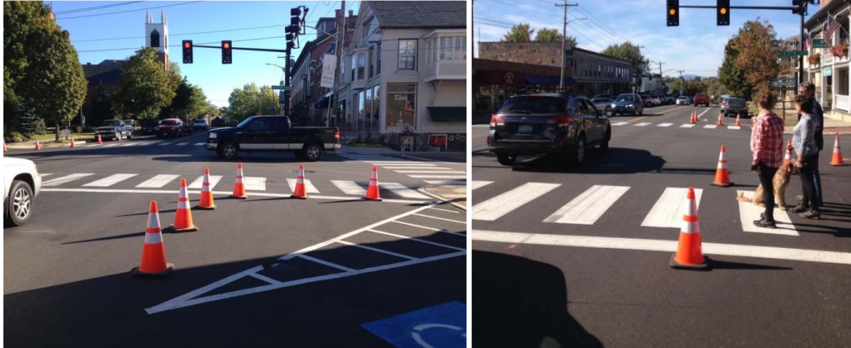
Figure 19: Traffic cones show how a curb extension would decrease traffic speeds while reducing pedestrian exposure to vehicles.
