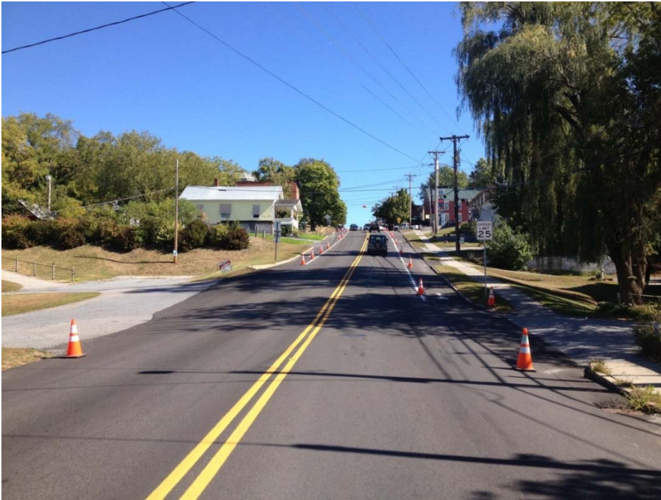
Figure 17: A 5' bike lane with a 2' buffer was demonstrated while maintaining 11' width for trucks in the adjacent travel lane.
