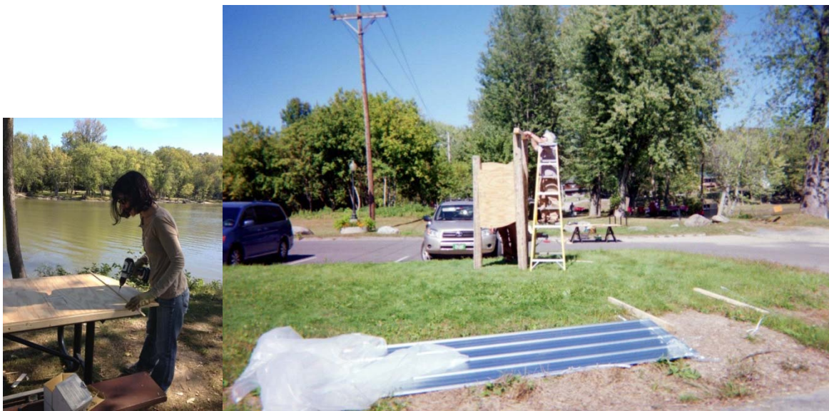
Figure 13: LandWorks and volunteers constructed the new kiosk in Falls Park.
