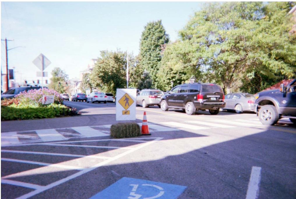
Figure 20: The hay bale and cone show how a curb extension would work to shorten pedestrian crossing distances and calm traffic.
